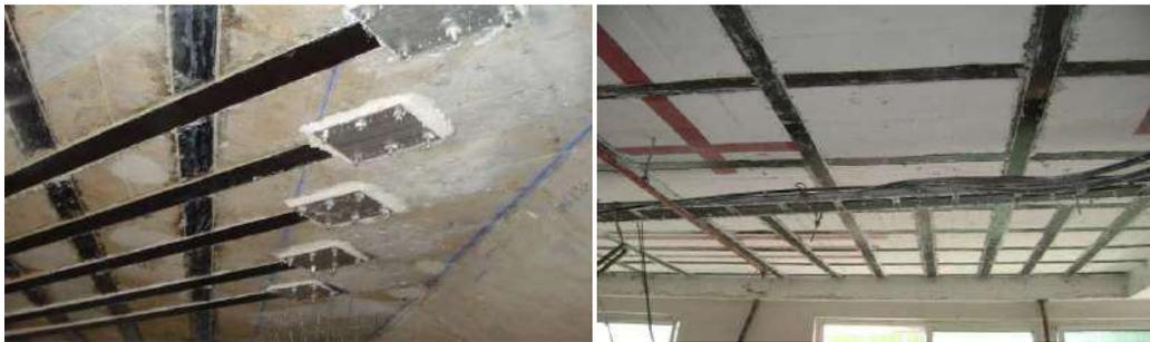
*Figure 7-18 Use of Laminates in for strengthening of slabs in a bridge and a building.*
