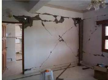
Infill panels to an reinforced concrete frame building acting as non-structural shear walls, provided stability to the overall frame – Bharasar, Gujrat
