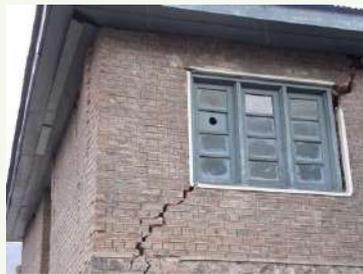
Uri town – Civil Defence Bldg.– Diagonal cracks in window openings and tilting of walls in Burnt Brick Cement Masonry wall, Kashmir, India.
